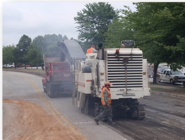
Milling an existing asphalt pavement.
