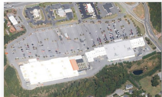
Asphalt pavement at a large shopping plaza.
