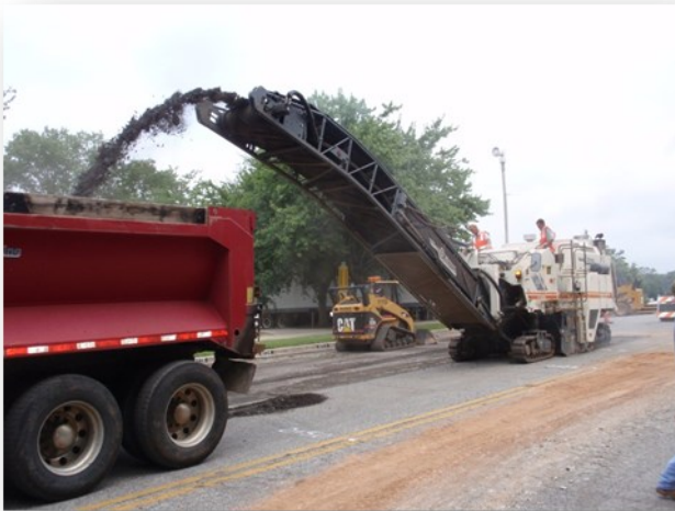
Removal of a controlled thickness of asphalt pavement using a milling machine.
