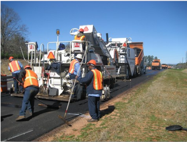
Placement of an asphalt surface course.
