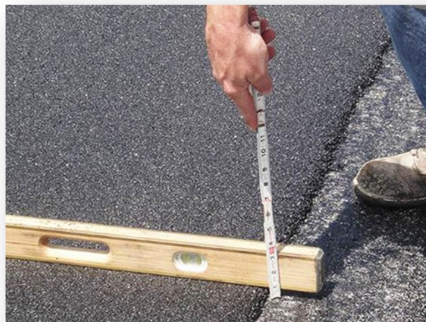
Thin lift asphalt overlay (thinlay).
