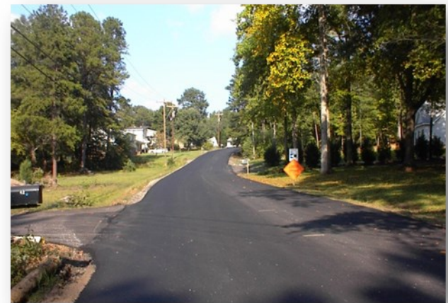
Asphalt pavement in a residential neighborhood.
