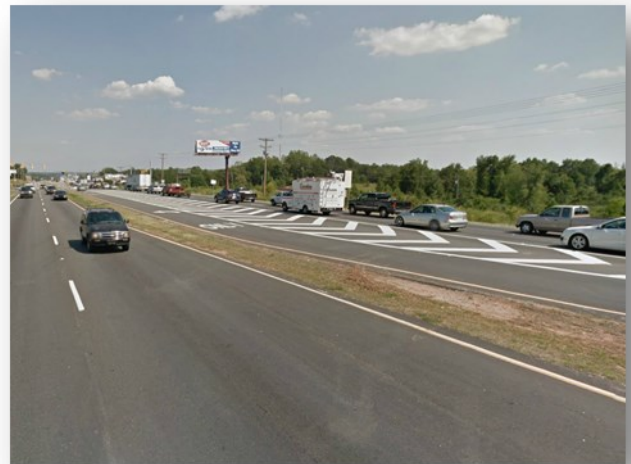
Asphalt pavement for a major arterial road.
