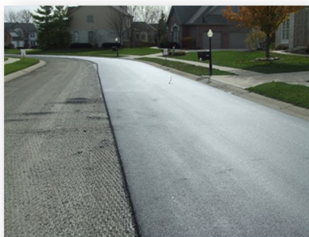
Newly placed asphalt overlay.
