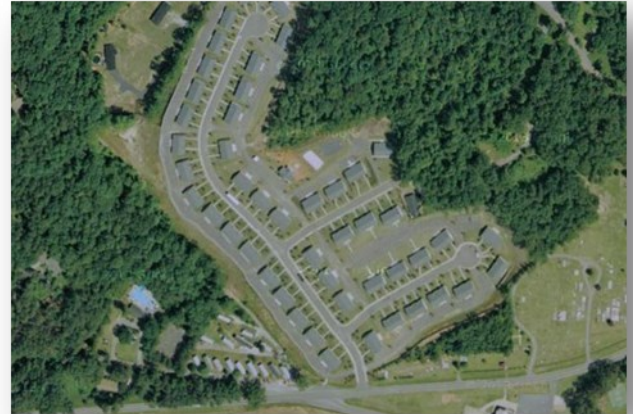
Asphalt pavement used for an apartment complex.
