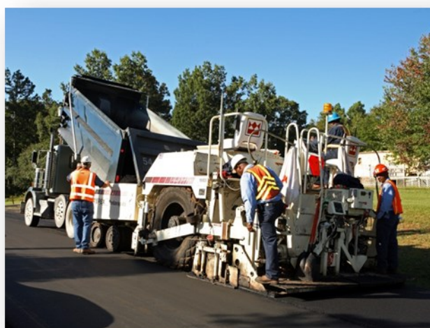
Placement of an asphalt overlay.
