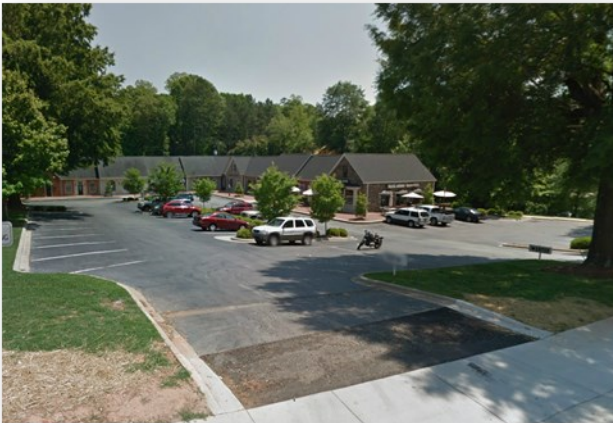
Asphalt parking lot serving a small plaza.
