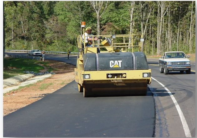
Compaction of an asphalt overlay.
