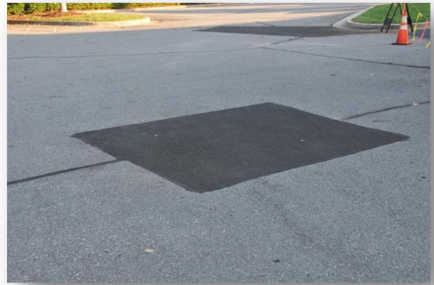
Finished full-depth patch.
