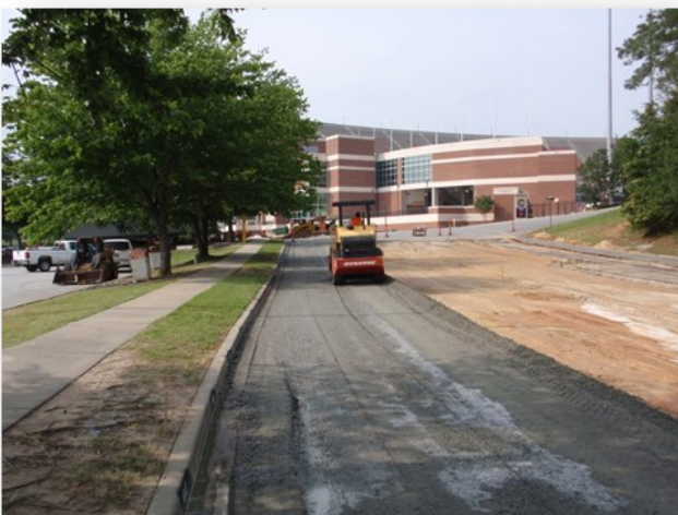
Preparation of subgrade and aggregate base course.
