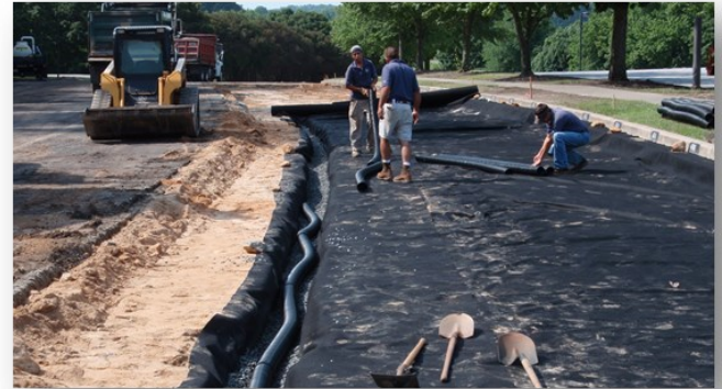
Installation of a pavement underdrain.
